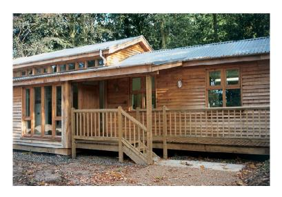
This is a new building of high ecological sustainability, using green oak felled on the site. The structure stands on legs, making only a light footprint on the ground. The interior is equipped with a suite of rooms, including a classroom and a laboratory. The How Hill Educational Trust enables children to study the freshwater life of the Norfolk Broads.
