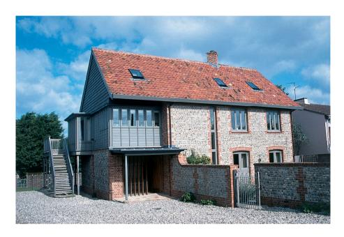
An imaginatively designed house on the coast at Brancaster. which has used local materials of brick, flint, and wood with extremely good detailing. The main living area is on the first floor, giving wonderful views of the marshes. creeks, and hills.
